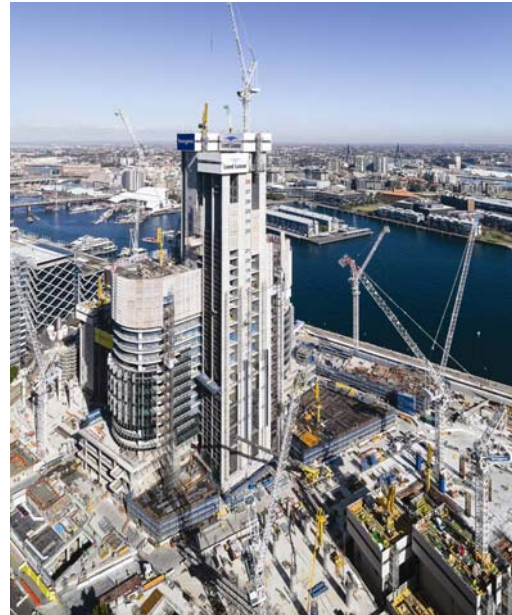
Barangaroo South Tower 2 under construction Source: Lend Lease
