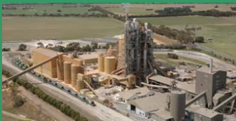
Wauron Ponds cement works
