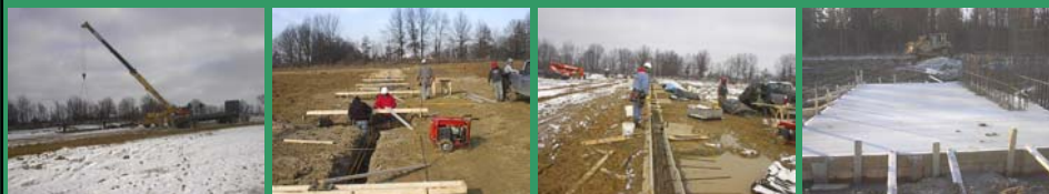
Indiana Brick Plant under construction
