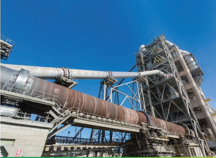
Boral Australia, Berrima Cement Works, NSW
